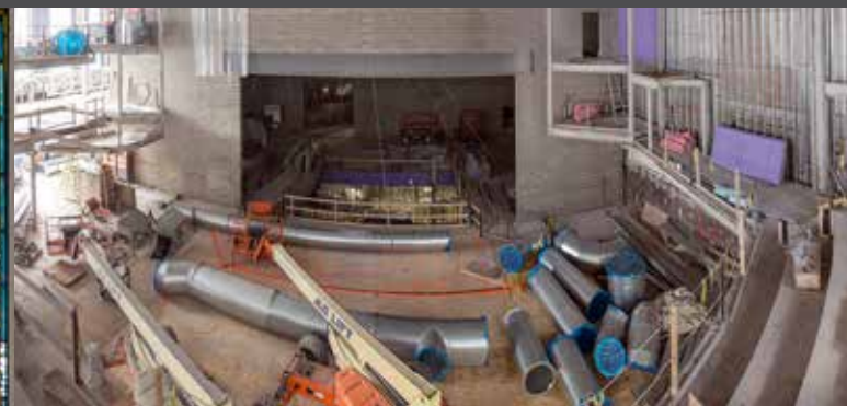
4,000 Peak number of weekly labor hours during construction
