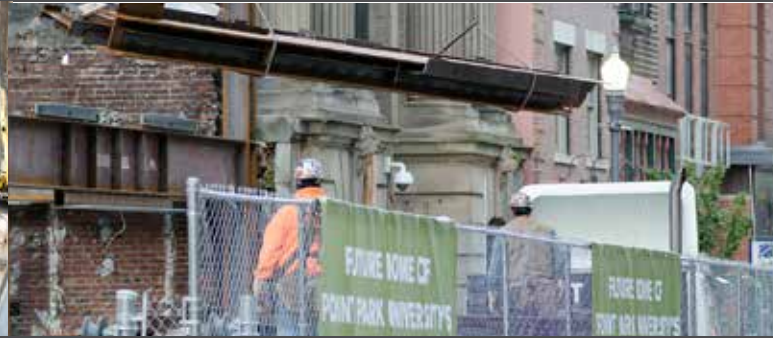
28 Months for construction
