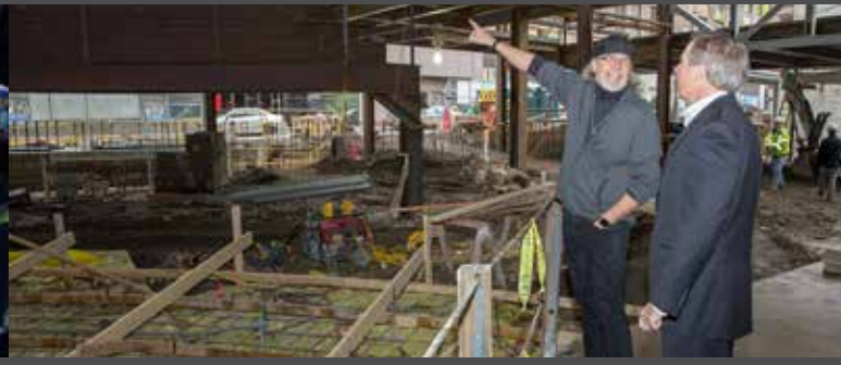
250,000 Feet of electrical conduit used throughout the building
