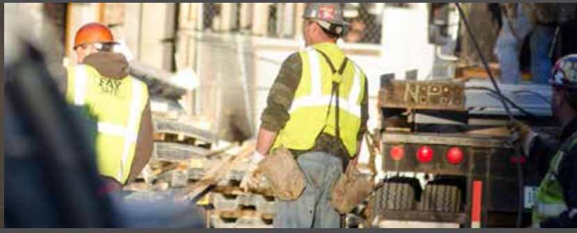
253 Total number of workers on the project
